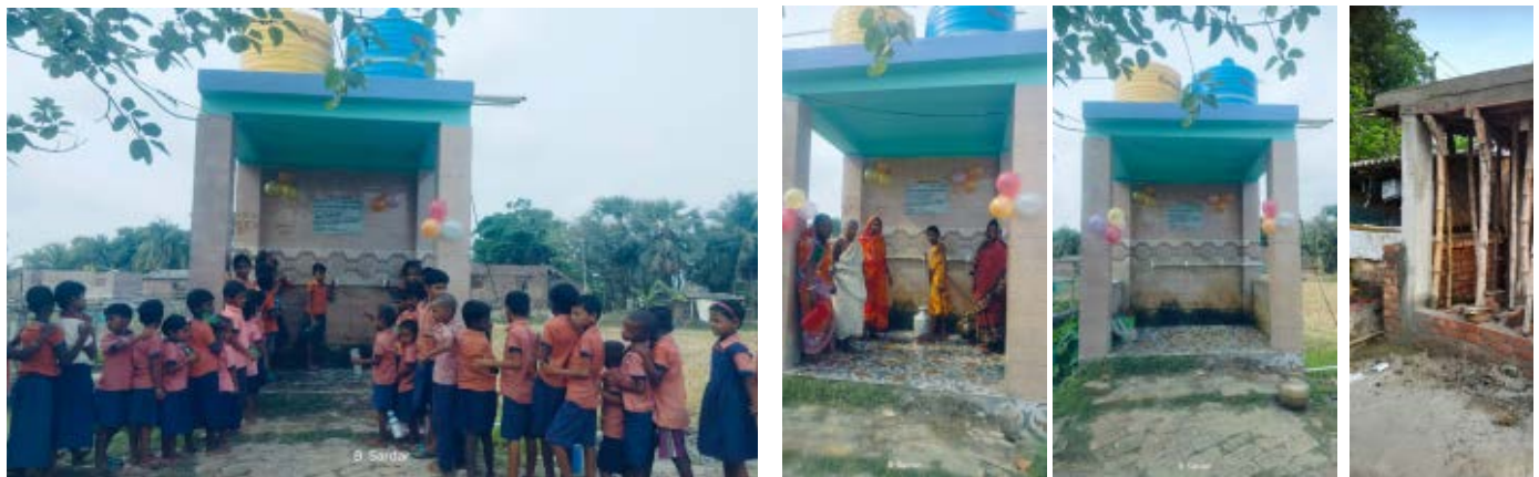
TUBE WELL # 193 at 4 No. Dakshin Garankati, Kultali, Sundarbans
